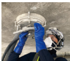
Concrete surface treatment using water-jetting
