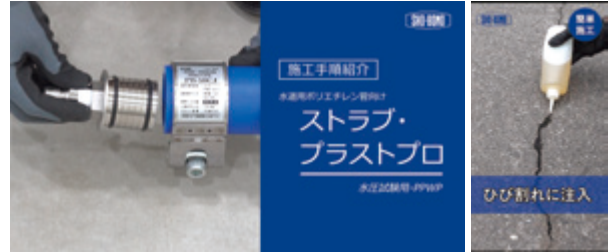
Video introducing our construction methods (SHO-BOND official YouTube channel)
