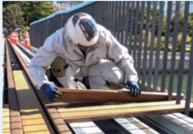
(3) Installation of wooden decking to surround the railway tracks
