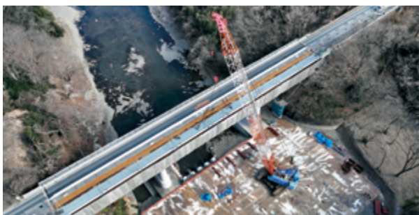
Superstructure widening work
