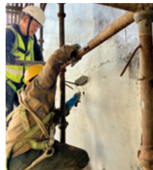
Trial construction in India
