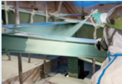
(1) Repainting work to recreate the bridge's original color during its use for transporting freight
