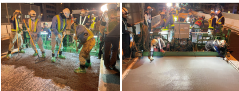
LSF trial construction on the Metropolitan Expressway
