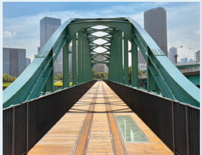
(3) Installation of wooden decking to surround the railway tracks
