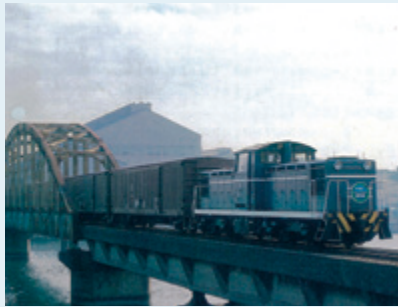
The bridge during its use for transporting freight (photo courtesy of Tokyo Port Promotion Association)
