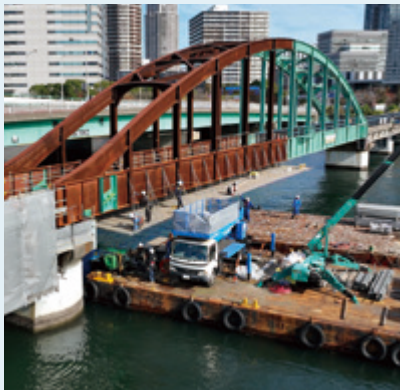
(1) Repainting work to recreate the bridge's original color during its use for transporting freight
