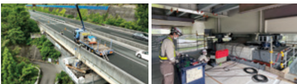
(Left) Construction work on a bridge in use. Passenger vehicles are passing in close proximity to the construction crane.
