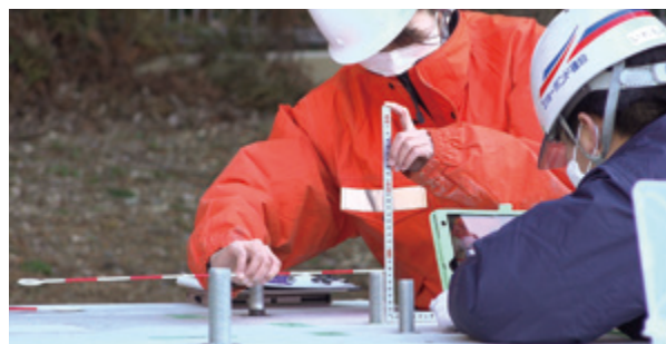
Practical training on anchor hole dimensional inspection and quality control
