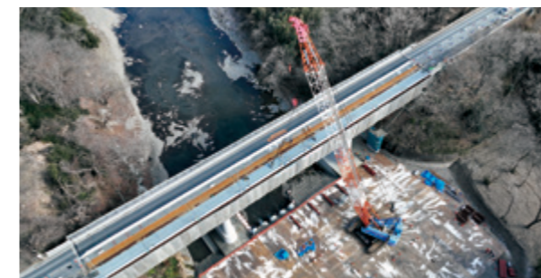
Superstructure widening work
