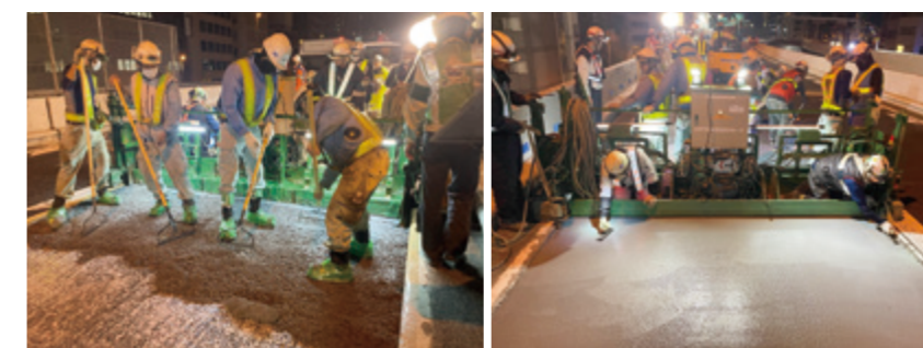
LSF trial construction on the Metropolitan Expressway
