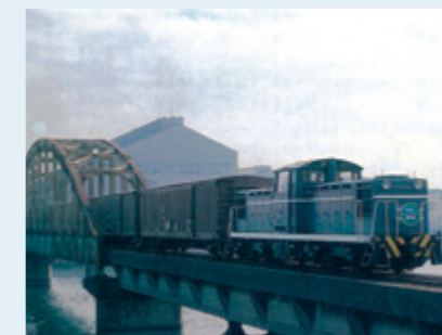
The bridge during its use for transporting freight (photo courtesy of Tokyo Port Promotion Association)
