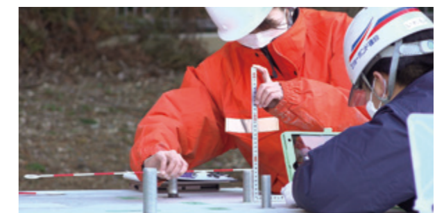
Practical training on anchor hole dimensional inspection and quality control
