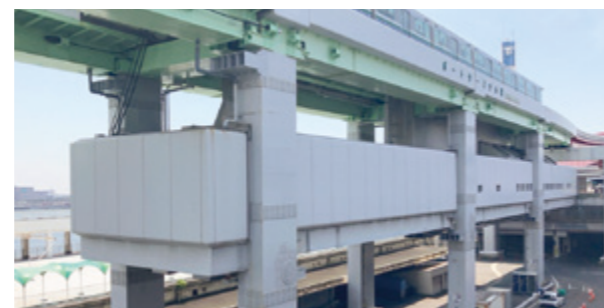
Railway construction project (completed seismic reinforcement of Kobe New Transit Port Island Line [PT Station and NK Station])
