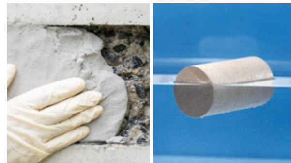
"L Putty" (left: repair work with L Putty, right: a lump of L Putty floating in water due to its light weight)
