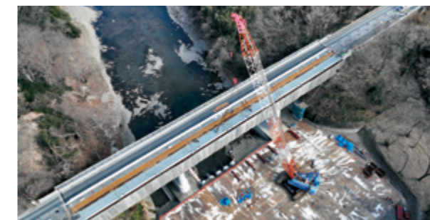
Superstructure widening work
