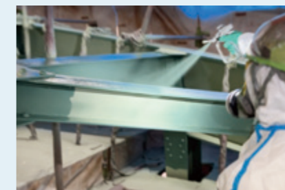
(1) Repainting work to recreate the bridge's original color during its use for transporting freight
