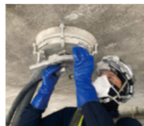
Concrete surface treatment using water-jetting
