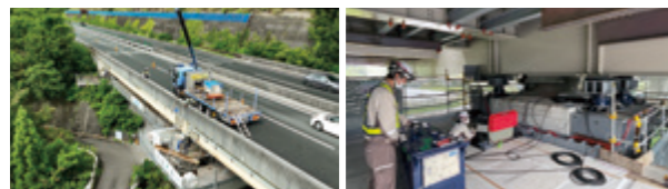
(Left) Construction work on a bridge in use. Passenger vehicles are passing in close proximity to the construction crane. (Right) Jacking up the superstructure. The in-use bridge girder is being lifted with jacks to replace the bearings.
