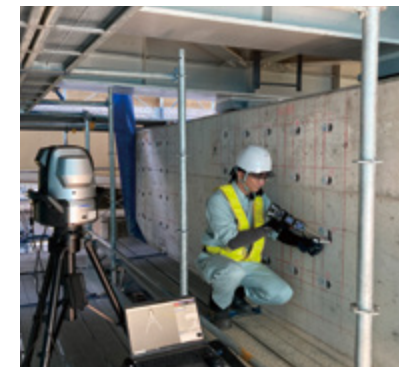
The status of measuring anchor bolt drilling positions using a 3D measuring instrument
