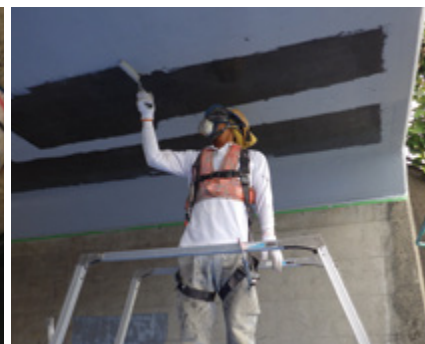
Spalling prevention using single-component water-based urethane resin
