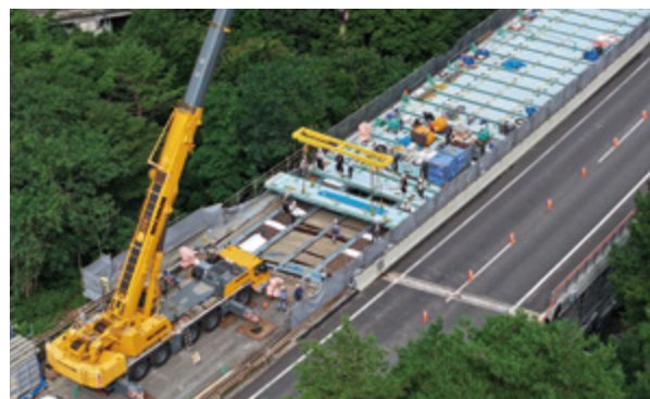
Replacement of deck slabs at Tengu Bridge
