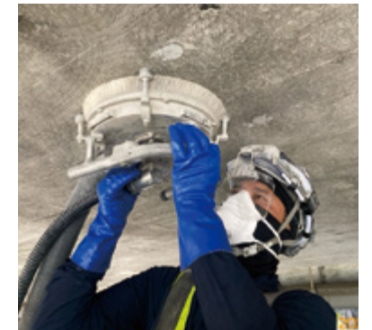
Surface preparation of concrete using water jet
