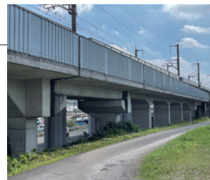
A railway concrete block wall reinforced using the Galette Sandwich Method
