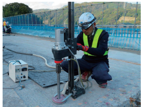
The use of high-frequency core drilling for anchor bolt holes
