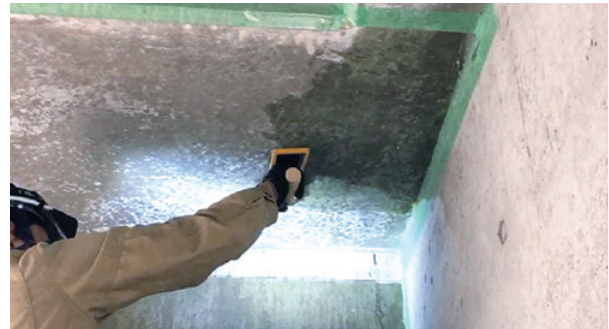
Application of SBLN GEL on a concrete structure
