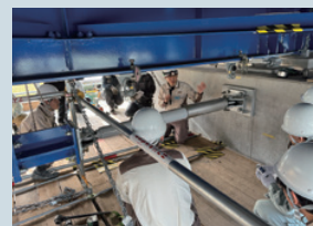
Practical training in installing seismic retrofitting equipment
