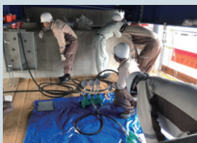
Practical training in jacking up bridges
