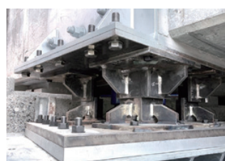
An installed jack featuring a movement restriction function
