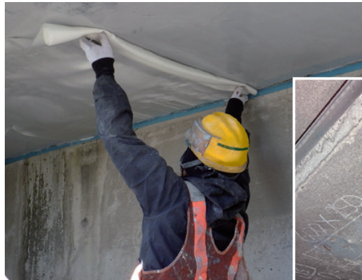
Applying a sheet to prevent chunks of concrete from breaking off and falling
