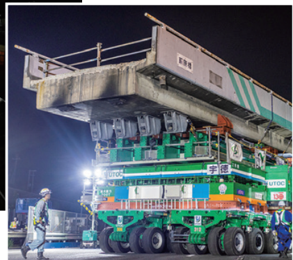
Removal of an expressway overpass bridge
