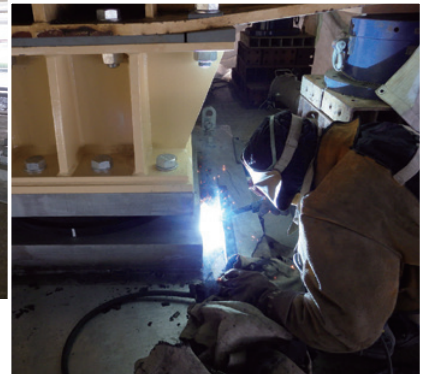
One step of the bridge-bearing replacement process
