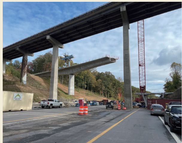
A Structural Technologies construction site
