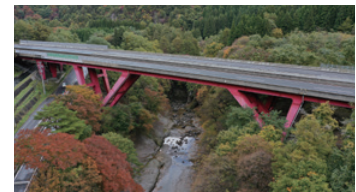
The Tengu Bridge on the Tohoku Expressway
