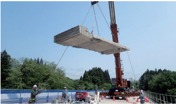
A construction site of the Expressway Renewal Project in 2018
