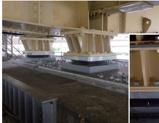
A bridge with new bearings in place
