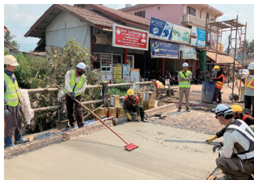
JICA trainees at the Technical Research Institute (above) and SHO-BOND engineers guiding a construction site in Laos (below)
