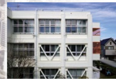
Buildings Seismic retrofitting
