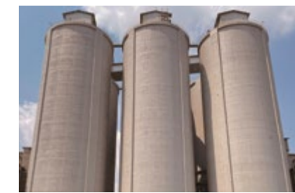
Silo Repair of wall surface degradation
