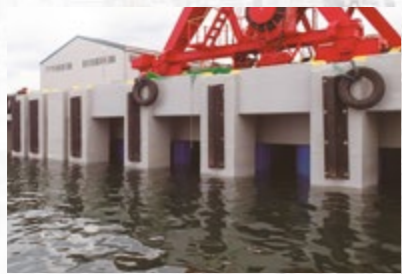
Harbor Quay Protection from salt damage Prevention of concrete degradation
