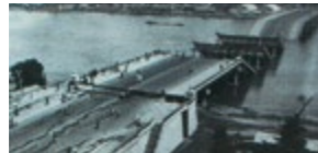
The Showa Ohashi Bridge in Niigata collapsed in 1964 during a powerful earthquake
