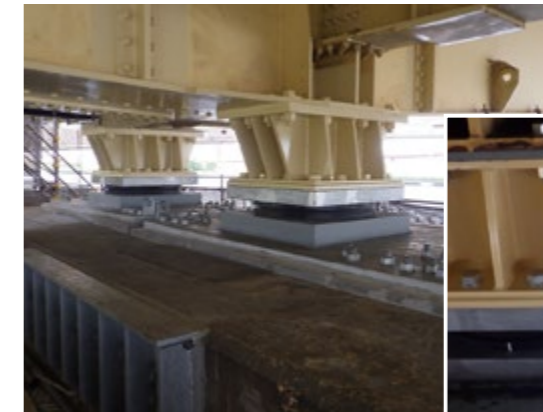
A bridge with new bearings in place
