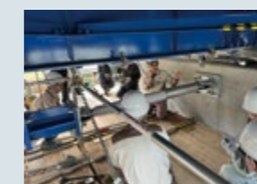
Practical training in installing seismic retrofitting equipment
