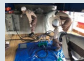
Practical training in jacking up bridges
