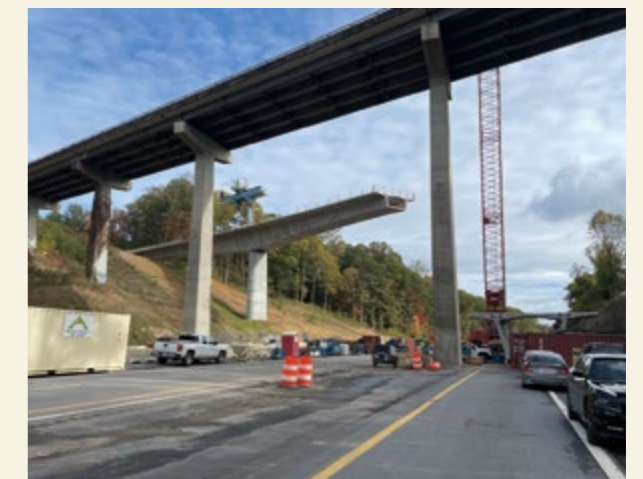
A Structural Technologies construction site
