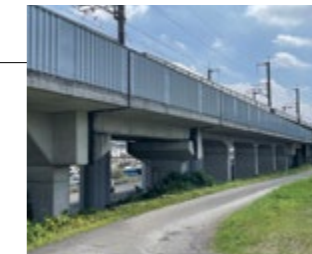
A railway concrete block wall reinforced using the Galette Sandwich Method
