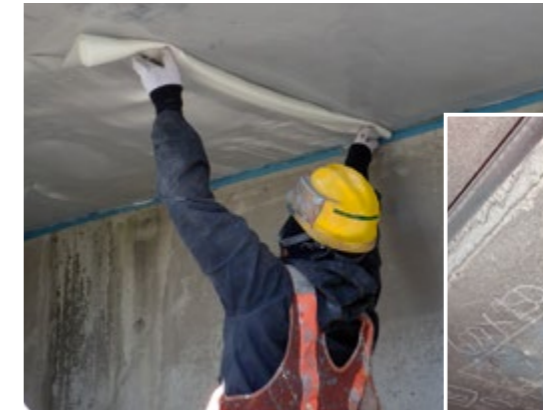
Applying a sheet to prevent chunks of concrete from breaking off and falling
