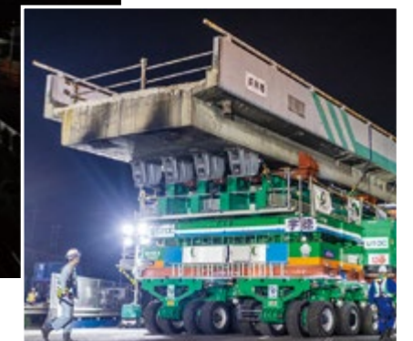
Removal of an expressway overpass bridge
