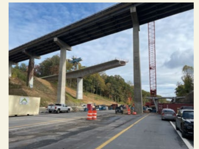
A Structural Technologies construction site
