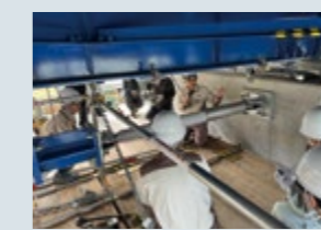
Practical training in installing seismic retrofitting equipment
