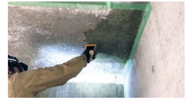
Application of SBLN GEL on a concrete structure
