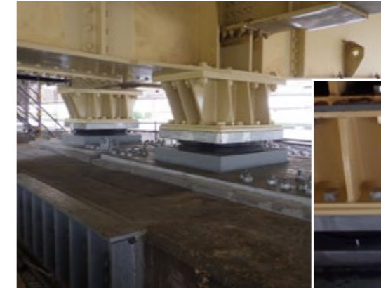
A bridge with new bearings in place
