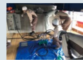
Practical training in jacking up bridges
