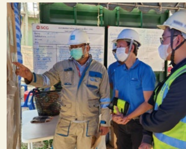
A construction site meeting
