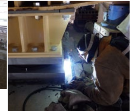
One step of the bridge-bearing replacement process
