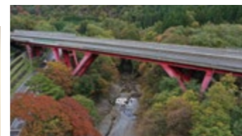
The Tengu Bridge on the Tohoku Expressway
