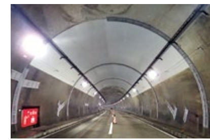
Tunnels Prevention of ceiling and wall spalling Stop groundwater leaks
