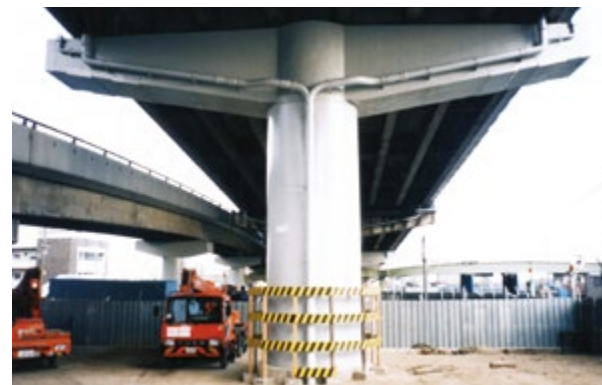
Piers of the expressway bridges reinforced shortly before the 1995 Kobe earthquake were not damaged by the powerful tremors
