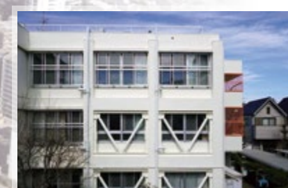
Buildings Seismic retrofitting
