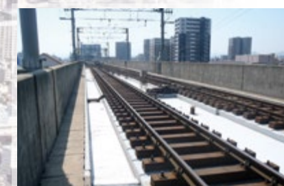
Railways Repair of damage at elevated railways Seismic retrofitting
