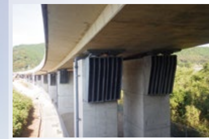
Bridges Seismic retrofitting Prevention of concrete degradation
