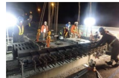
Road structures Repair of expansion joints Noise reduction
