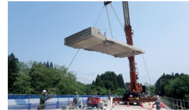
A construction site of the Expressway Renewal Project in 2018
