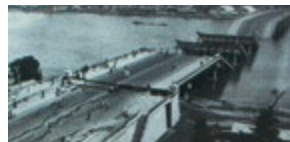
The Showa Ohashi Bridge in Niigata collapsed in 1964 during a powerful earthquake
