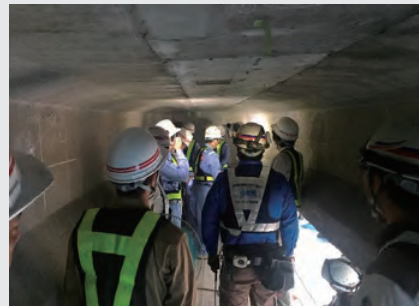
An inspection by a Bridge Doctor
