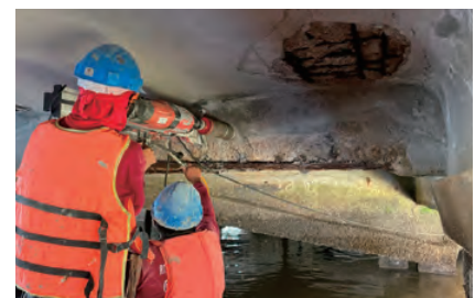
A port repair site in Thailand
