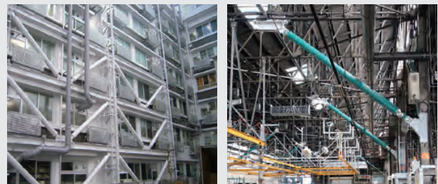
Reinforcement work in progress
