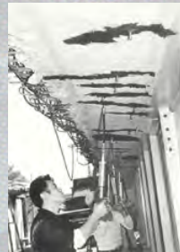
◀ The state of the cracks viewed from directly below the deck slabs
