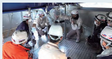
Practical training in installing bridge fall prevention equipment (at the training bridge)
