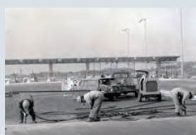
1967 Installation of the Cut-off Joint at the Tomei Expressway Nagoya Interchange
