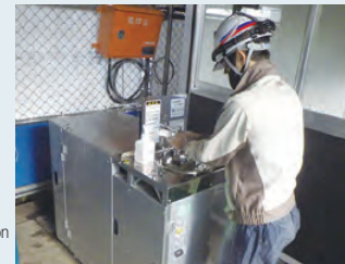
Circulation-type hand wash station installed at a site
