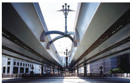
1991 Exterior work at the bridge over Nihonbashi
