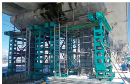
2011 Repairing Tohoku Shinkansen columns damaged by the Great East Japan Earthquake
