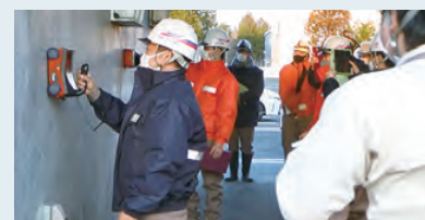
Practical training in finding rebars location
