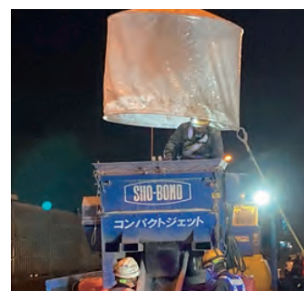
Construction site (CPJ-L)
