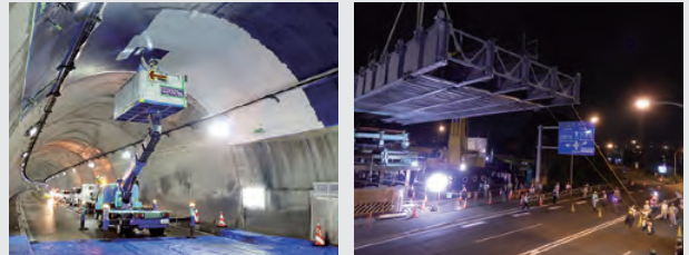
Renewal work underway
