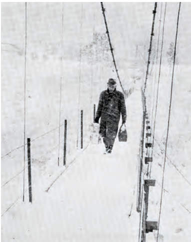
1961 Founder Akira Ueda transports building materials to a dam construction site during a blizzard
