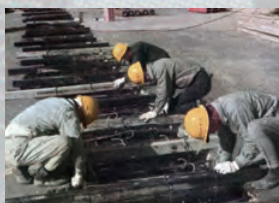
▲ Setting up concrete forms
