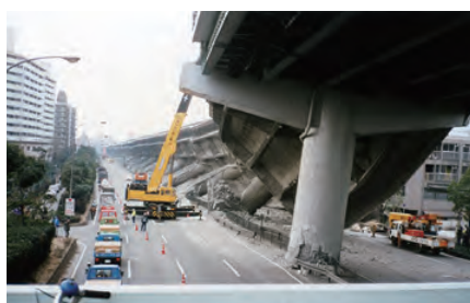
1995 A section of the Hanshin Expressway destroyed by the Great Hanshin-Awaji Earthquake
