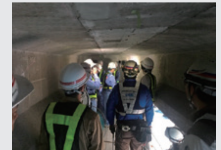
An inspection by a Bridge Doctor
