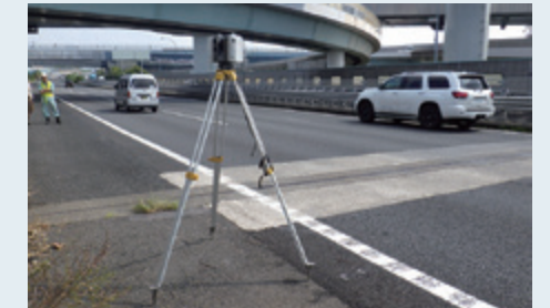
Structure measurement using a 3D scanner
