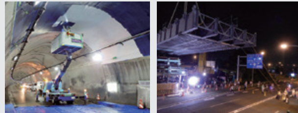
Renewal work underway
