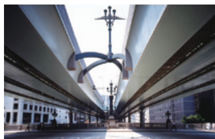
1991 Exterior work at the bridge over Nihonbashi
