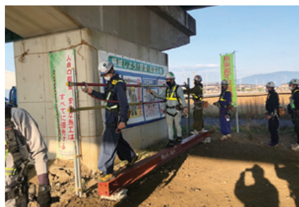
On-site safety training
