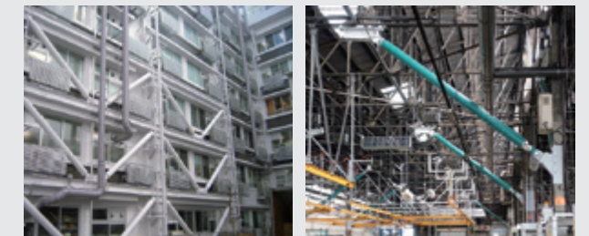
Reinforcement work in progress
