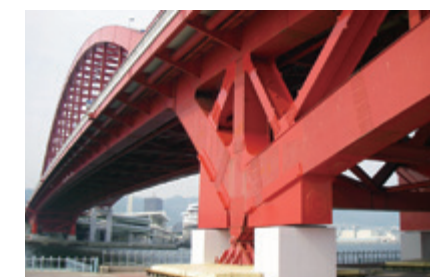
2011 SHO-BOND's work at the Kobe Ohashi Bridge received a Technology Award from the Japan Society of Civil Engineers Kansai Branch
