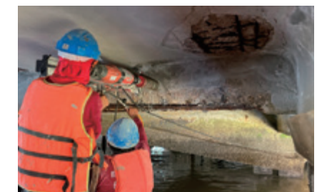
A port repair site in Thailand
