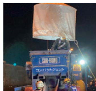
Construction site (CPJ-L)
