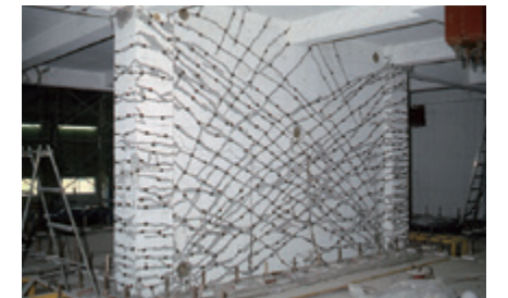
1981 The SHO-BOND BICS (Balloon Injection for Concrete Structures) Method for repairing cracks in concrete was used at the Japan-U.S. large earthquake resistance experiment at the Building Research Institute of the Ministry of Construction.
