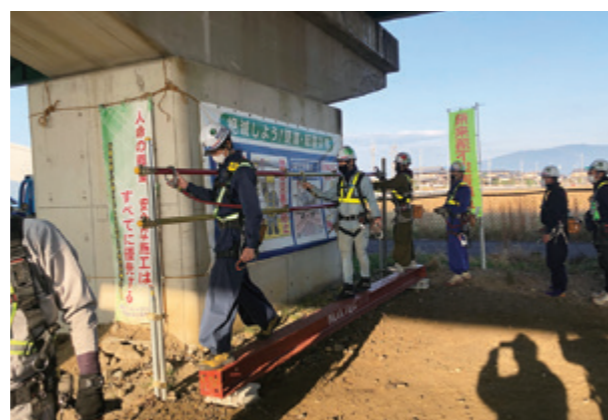
On-site safety training
