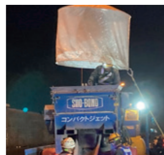
Construction site (CPJ-L)
