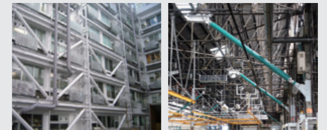
Reinforcement work in progress
