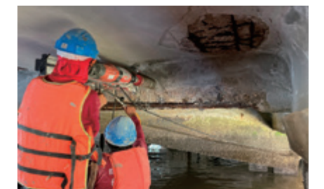
A port repair site in Thailand
