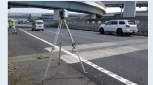
Structure measurement using a 3D scanner
