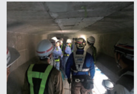
An inspection by a Bridge Doctor
