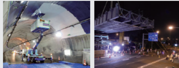
Renewal work underway
