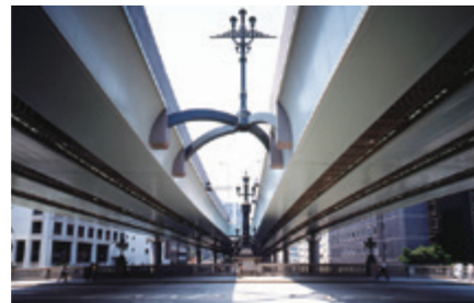
1991 Exterior work at the bridge over Nihonbashi
