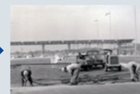
1967 Installation of the Cut-off Joint at the Tomei Expressway Nagoya Interchange
