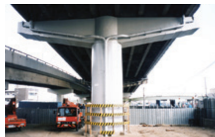
1995 Expressway columns reinforced shortly before the earthquake were intact
