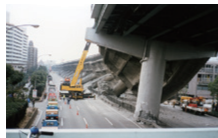
1995 A section of the Hanshin Expressway destroyed by the Great Hanshin-Awaji Earthquake
